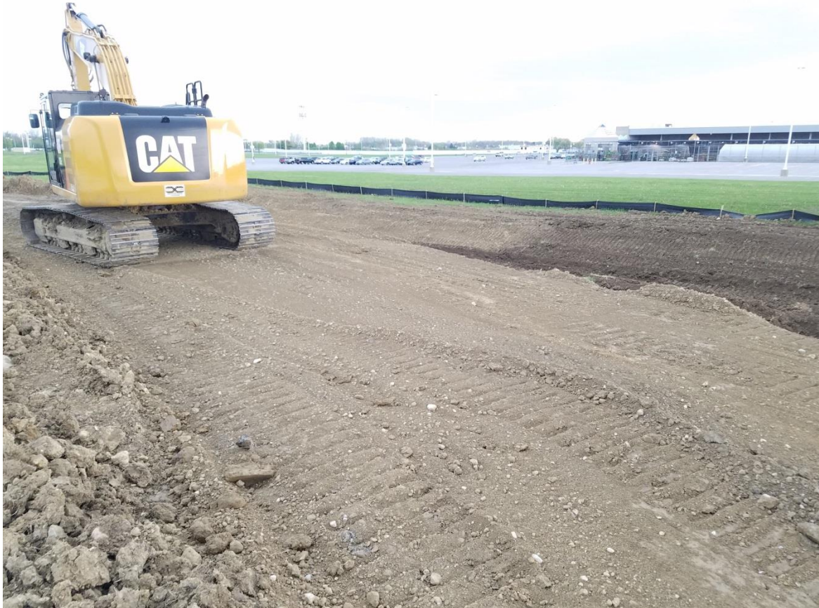
Project Site on May 3, 2018 looking north east showing the new access drive.
