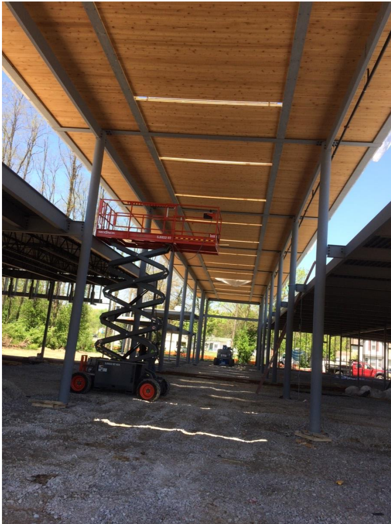
Project Site on May 3, 2018 with the completed wood roof deck for the Concourse.
