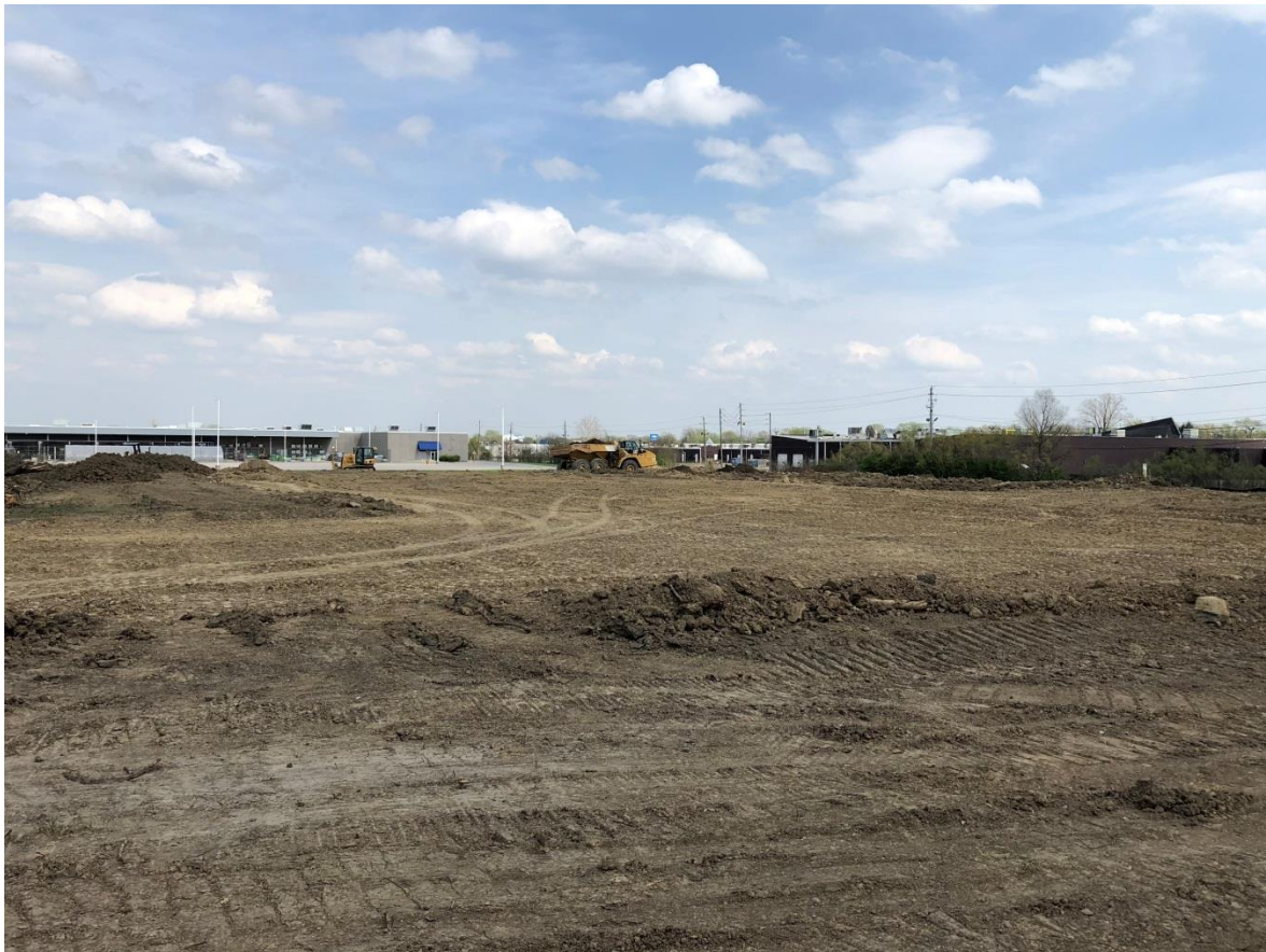
Project Site on May 3, 2018 View from the west showing the building pad.
