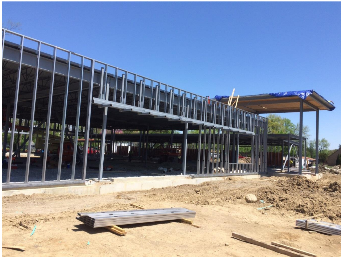
Project Site on May 8, 2018 View from the southwest showing the form of the building and the metal stud framing of south exterior wall.
